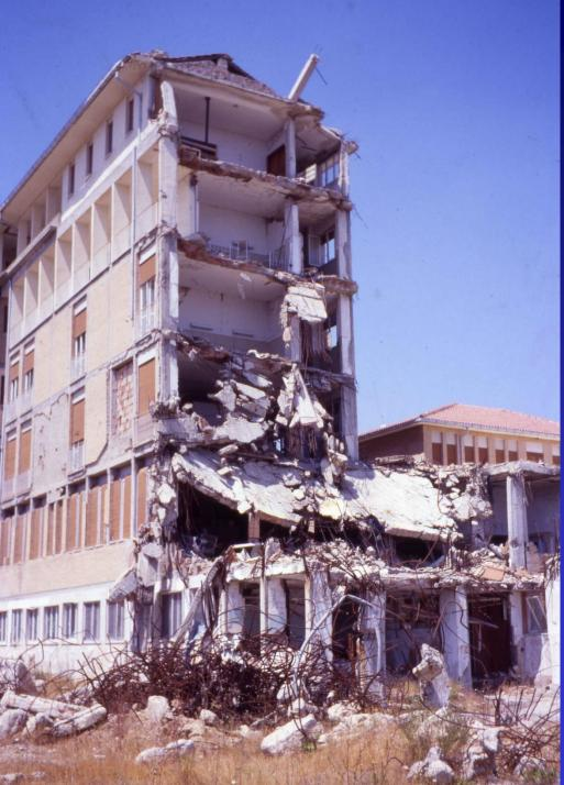
Compared to the original plans, this hospital lacked more than 500 concrete beams. In the earthquake, there was mass mortality in the maternity wing.
